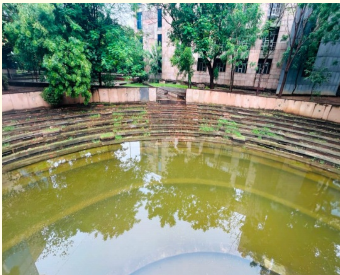
Rainwater harvesting at FDDI, Ankleshwar Campus
